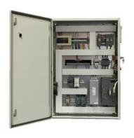
Bidirectional Energy Storage Inverter Photovoltaic on/off Grid
