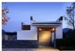
Household Energy Storage
